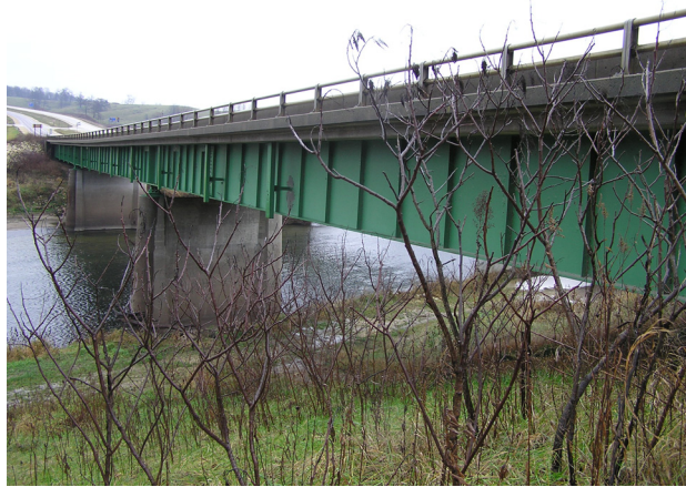
a. Photograph of the US151 bridge
