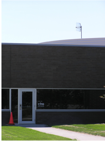
Figure 4.7. Antenna mounted on the rooftop of the ISU BEC.
