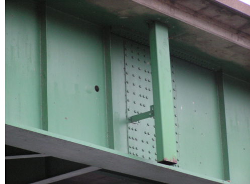
b. Photograph of web splice retrofit
