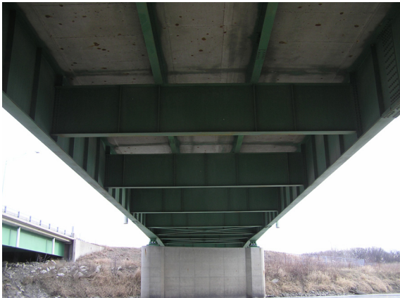
b. Girders, stringers, floor beams, and stiffeners
